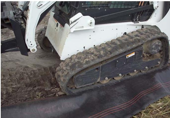
After the fence has been sliced in, use the tractor or loader to drive over the sliced trench and compact the soil. This will lock the fabric in place. For a proper installation, the soil should be compacted before the posts are installed.
